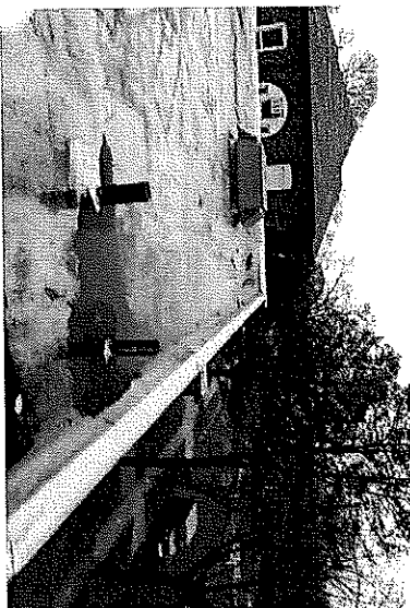
This is an asphalt built-up roof over an older asphalt built-up roof.
